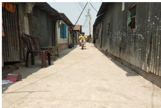
Footpath constructed at Rail Colony CDC under 2019 SIF grant
